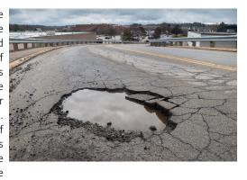
road, pieces of the pavement weaken, which causes the material to break down from the weight, creating the pothole.
